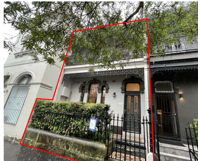
Pitt Street - eastern facade
